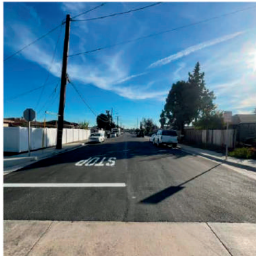
Bottom left photo: completion of Lorna St. (South of Stanford Ave.)
