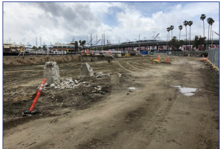
Excavation Behind Sea Wall
