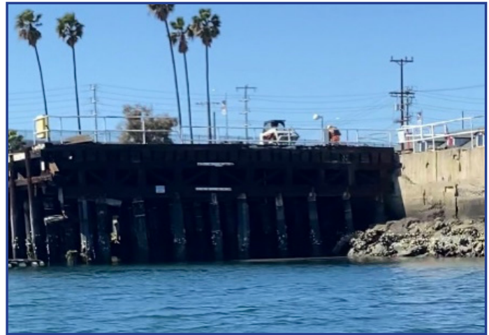
Breaking AC Over Timber Wharf
