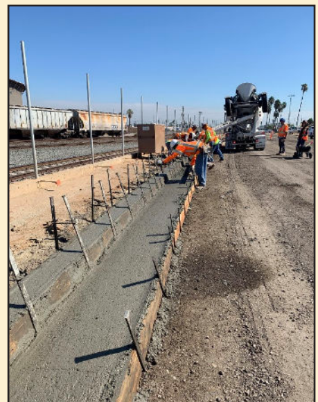
Pouring curb and gutter along new Water St.
