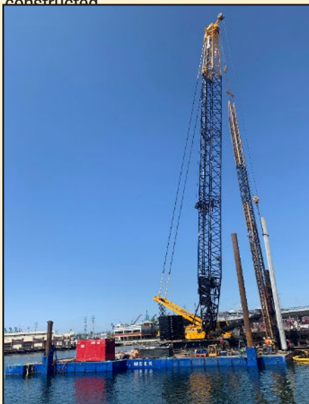
Installing octagonal concrete piles.
