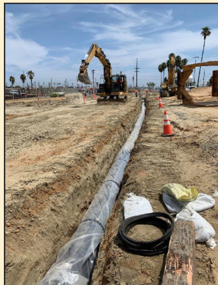
Installing 16" ductile iron waterline.
