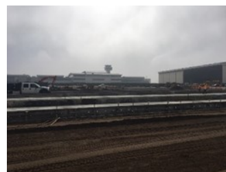
Phase 9 Tunnel August 3, 2020
