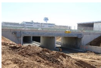
Phase 9 Tunnel April 15, 2020
