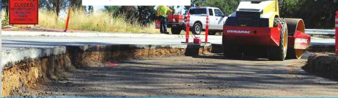
(Below) Compacting base material on Imperial Highway on-ramp.
